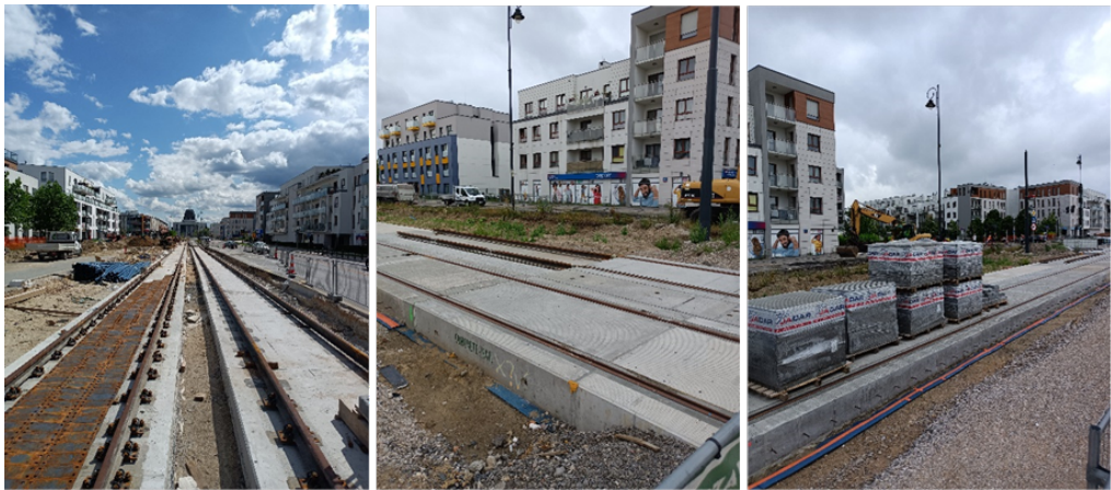
Fig. 2. Tram line under construction in 2024. Source: author's archive
