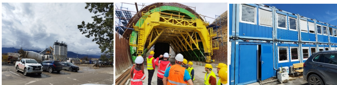
Fig. 5. Main basis, concrete junction, and formwork for open tunnel construction
