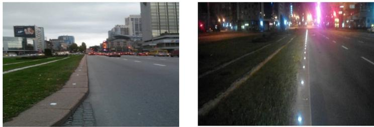
Fig. 13. Experimental implementation of retro-reflective elements
